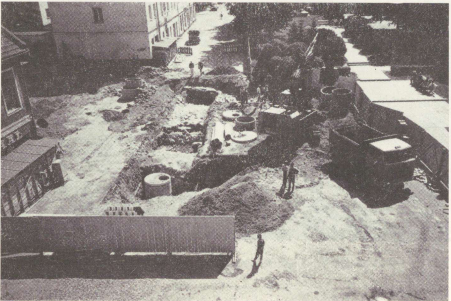
2. Viljandi. General view of the excavation area (from the north).
