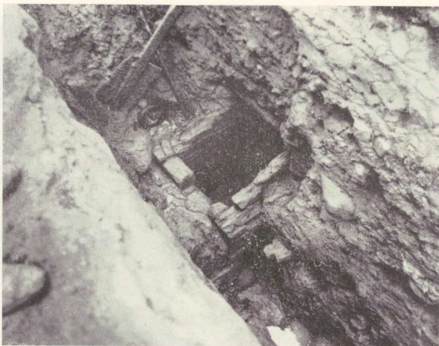
1. Tartu, K uutri Street. Settling well. View from the north.
