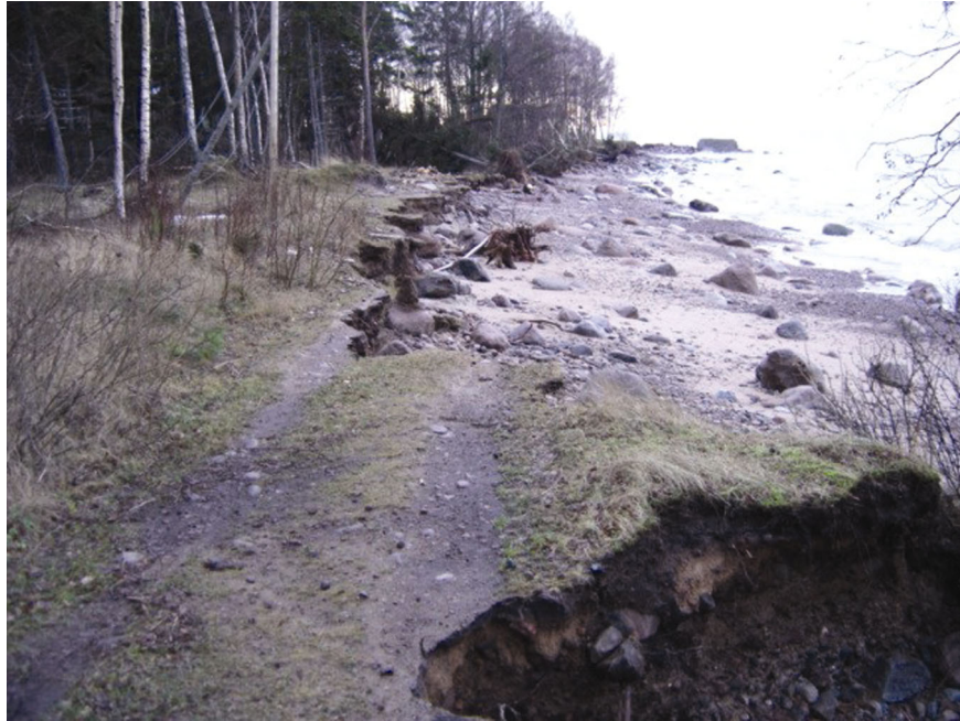
Fig. 2. The damage to the Aegna Island coast after the storm in January 2005 (Photo by H. Udusaar).
