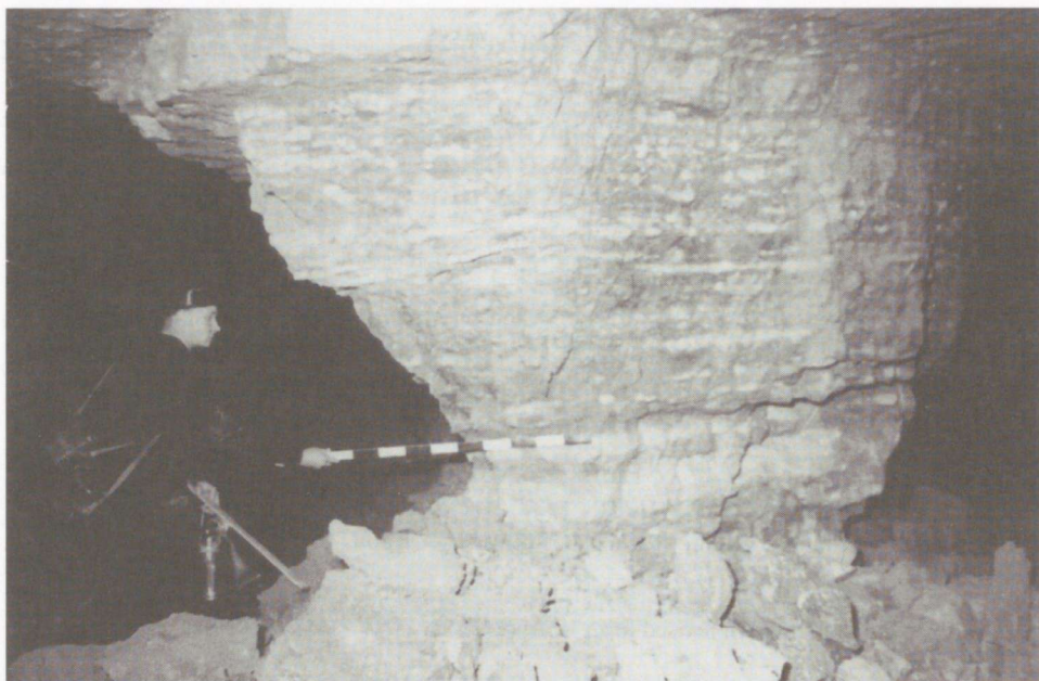
Fig. 1. Failed pillar in a collapsed room of the Ahtme mine in April 1965.
