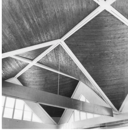
Fig. 4. Interior of a composite timber shell.
