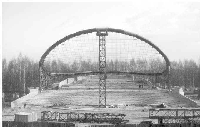
Fig. 5. Erection of the song festival tribune in Tartu.
