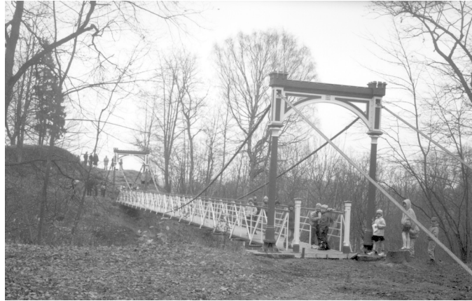
Fig. 6. Suspension footbridge in Viljandi.
