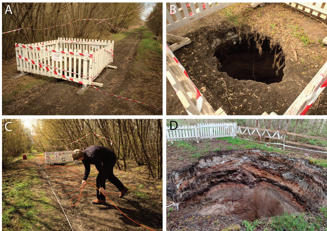
Fig. 3. A, B – studied sinkhole on 21.04.2021. C – array of the ERT profile near the sinkhole. D – sinkhole after one year on 12.05.2022. Note that after a year, the entire overhanging cover of the sinkhole where the ERT profiles were located has collapsed, and the sinkhole is almost as wide as the road.
