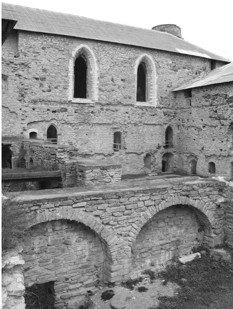
Fig. 6. View from room 2 to northeast. Foreground: reconstructed north wall of room 2. Background: south exterior of the church with traces of the two-storey cloister.
