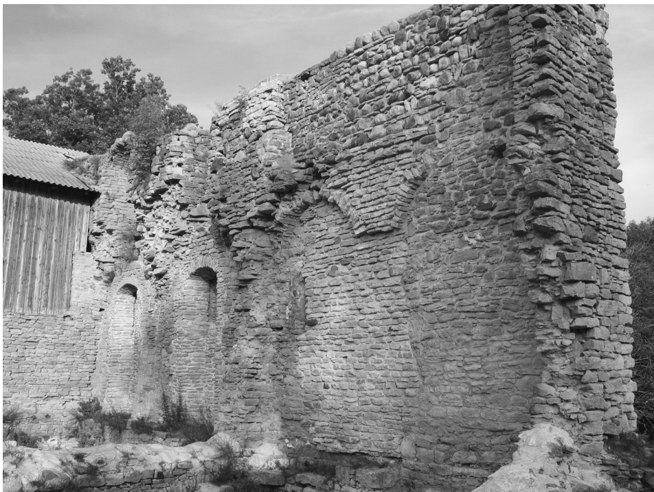
Fig. 7. Inside of the outer wall of the main storey of the southern wing.
