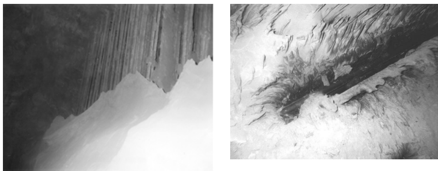
Fig. 6. Condition of boiler surfaces after 25 running days without sonic cleaning: a) superheater after 25 running days without sonic cleaning; b) economizer after 25 running days without sonic cleaning
