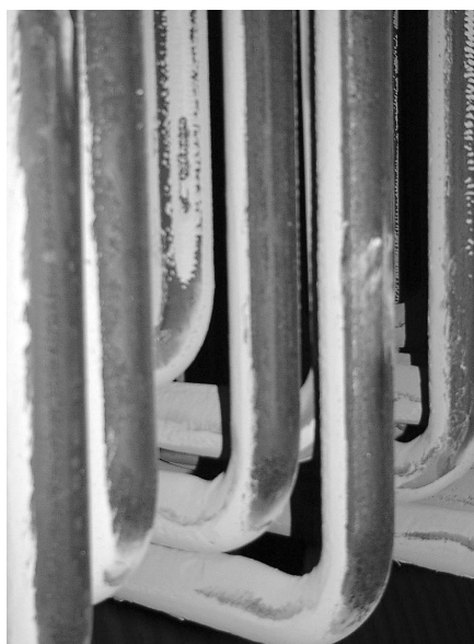
Fig. 6. Photos of superheater tubes: a – SH1B rear side; b – SH1A front side
