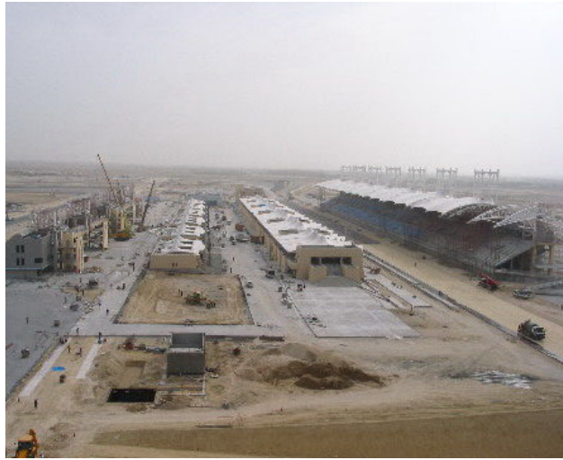
Figure 7. Bahrain FORMULA-1 Circuit project under construction.
