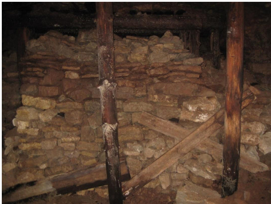
Fig. 4. Hand-mined area after oil shale extraction: limestone placed in the limestone wall (Kohtla Mining Museum) [16].
