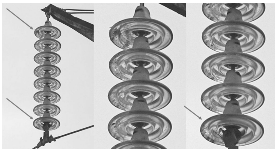
Fig. 12. Bird excrement imprints on glass insulator string (L178) (photo by V. Milt).
