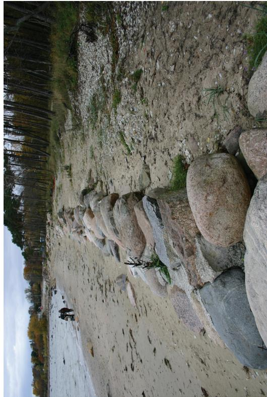
**Photo 3.** Remnants of the revetment originally constructed at the dune toe at the north end of Pirita Beach at the beginning of the 1980s. Photo by A. Kask.
