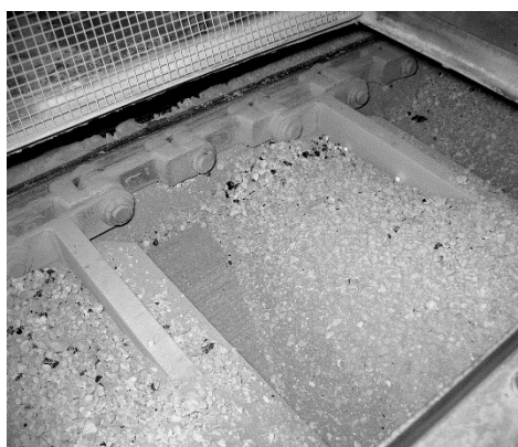
Fig. 5. Coal pieces still burning on the bottom ash conveyor.
