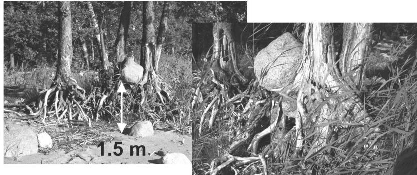
Fig. 7. Area of active erosion to the north of the Ust-Luga port terminal.
